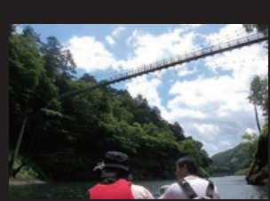
Mikaeri Suspension Bridge
