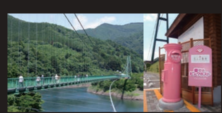
Momijidani Suspension Bridge
